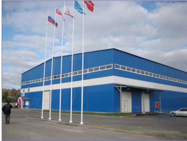
Exterior of Plant
